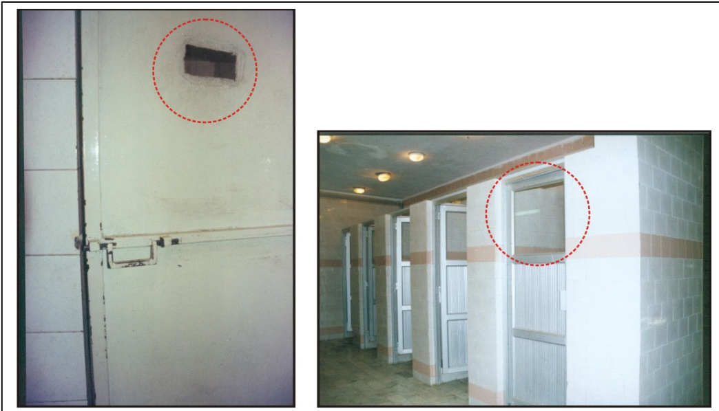
Figure 6: Due to the mentioned abuses, the restrooms especially male services often had a small window on the top of door where the guard could see the interior if there was a long occupancy.
