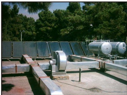
Figure 13: Solar water heater
