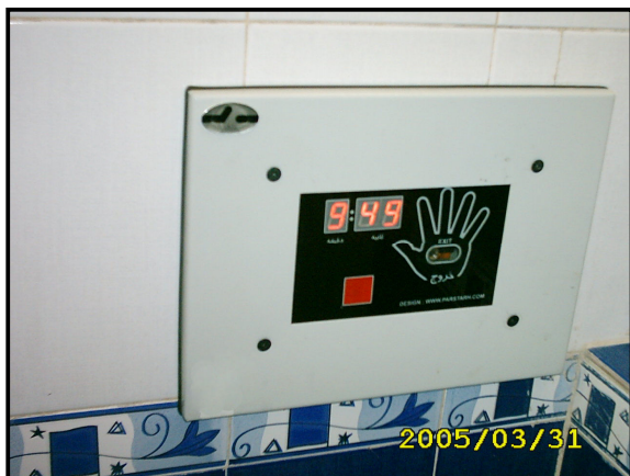
Figure 10: Internal count down timer and exit switch
