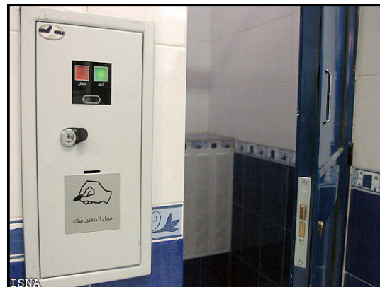
Figure 9: Smart entrance system
